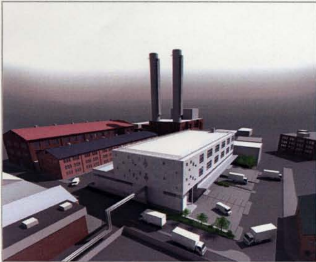
New Perry Avenue Building
